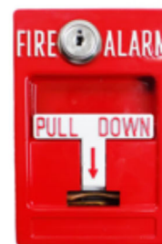
MANUAL PULL STATION
