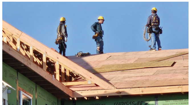
Roof Work Underway
