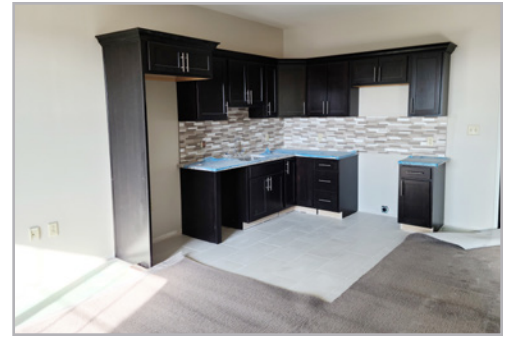
Backsplash & flooring installed in all apartments
