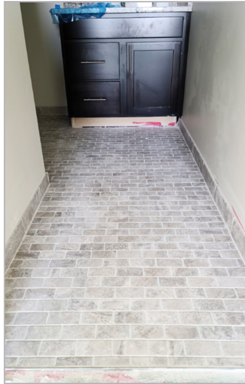
Tile installed in bathroom
