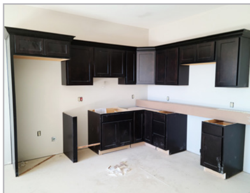
Cabinets being installed in IL apartments
