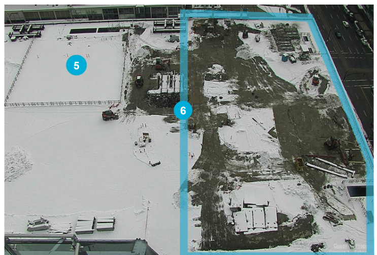
5 Opening in building for circular vehicle ramp
