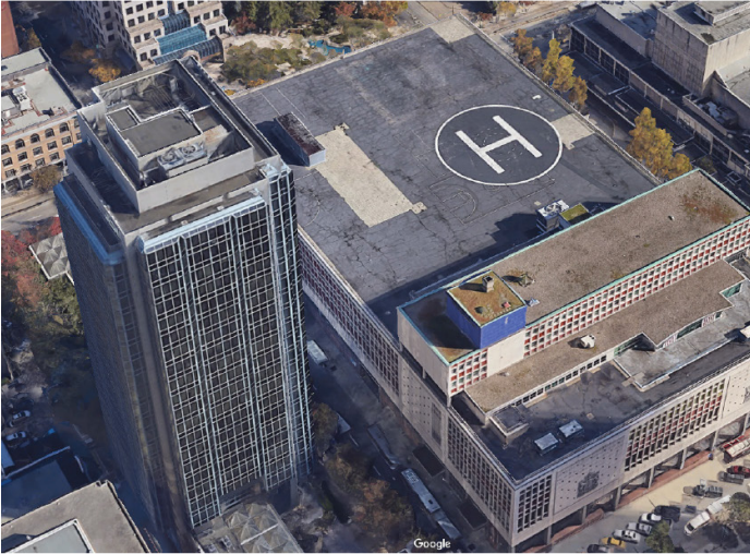
Canada Post building before construction
